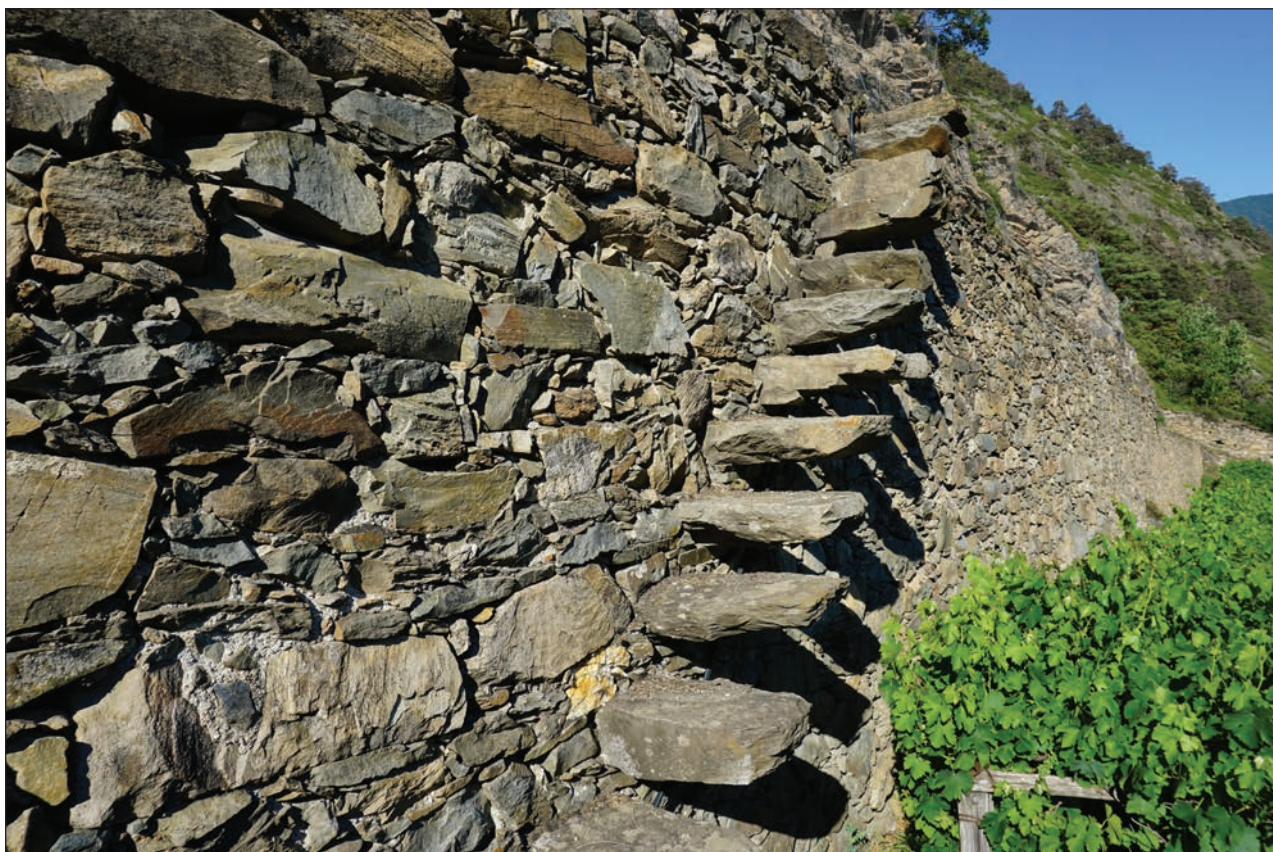
Figure 10: Stone ladder between vineyard terraces in Morgex area (Source: IAR, Aosta).
