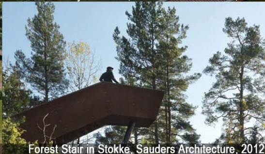
Forest Stair in Stokke, Sauders Architecture, 2012
