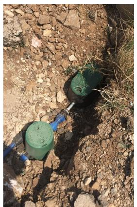
Figure 2: Testing of Water Network & Installation of House Connections
